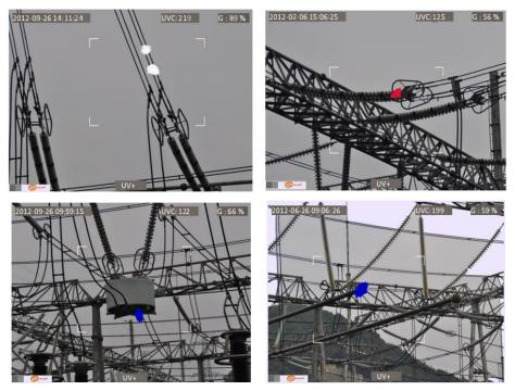
Fig. 5-8. Corona discharge in real power grids.
